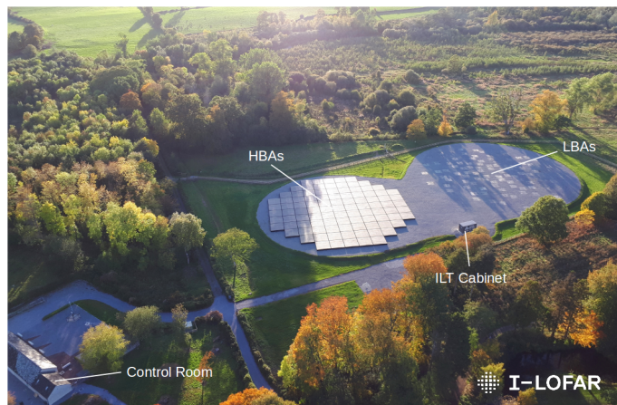
Fig. 1: The Irish Low-Frequency Array station IE613 (I-LOFAR) at Birr Castle, County Offaly. Coaxial cables are used to transport data from the Low Band Antennas (LBAs) and High Band Antennas (HBAs) to the ILT Cabinet (center right), where it is amplified, filtered, and digitalised. Data is sent in international mode at a speed of \sim 3.2 Gbps to Groningen, Netherlands. In the I-LOFAR Control Room, data is processed using REALTA in local mode (bottom left) (Murphy et al. 2021).
